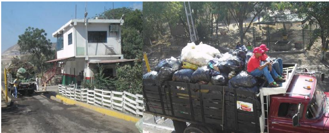
Image 8. Pictures of the Pavia landfill administrative facilities, and entrance of waste collection vehicle unit with mixed waste. (Rosell, February, 2011).
