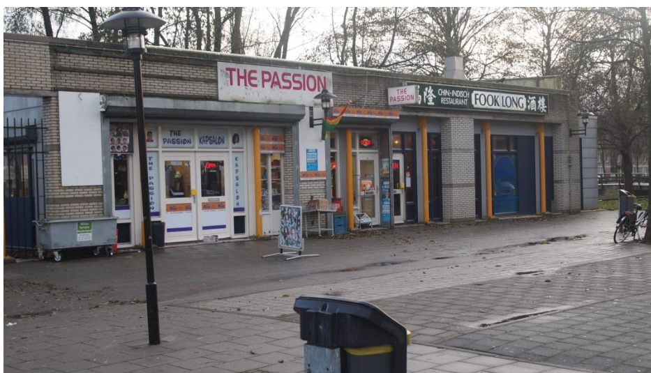
Figure 6.12: Venserpolder shops Source author
