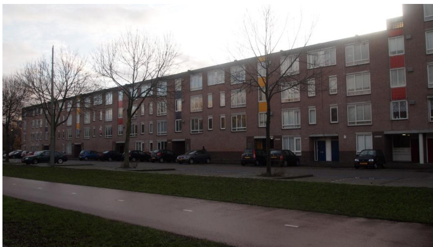
Figure 6.13: Venserpolder facade Source author
