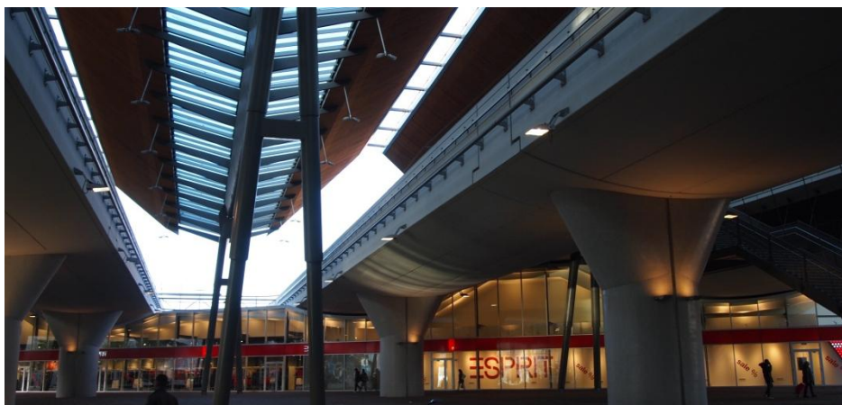
Figure 6.5: Bijlmer Metro Station Source author
