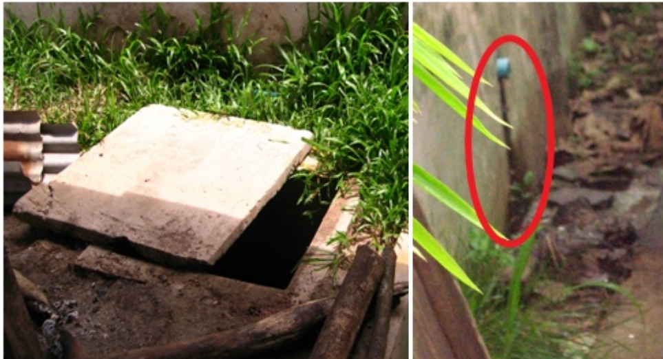
Figure 11: Sewage collected by septic tanks and open ditches.
