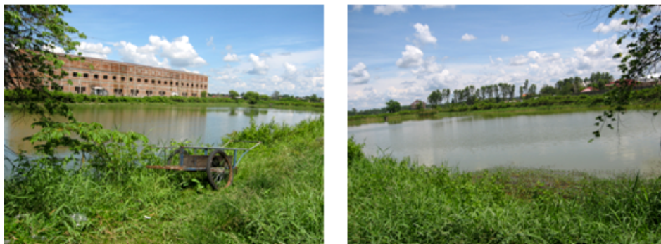
Figure 15: Construction sites and buildings near the facultative lagoons
