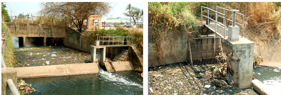
Figure 13: Water intake of EU ponds. Water dam and bar screen are built to trap large waste (with permission of Drs Lacoursière and Vought).
