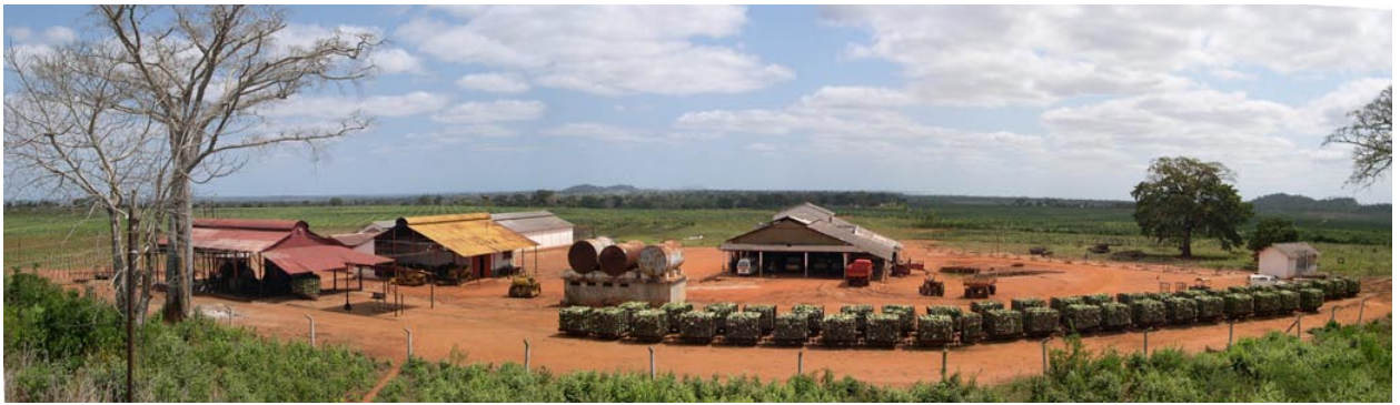
Figure 3. View over the Ramiane sisal plantation illustrating the flat topography of the area.
