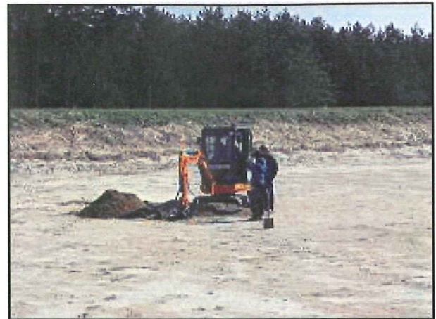
Fig. 7. Digging of profile C in basin no. 207.
