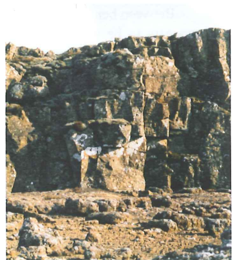
Fig. 18. Less than 50m westward from Fig. 17 the vertical walls give way to a clear fault scarp. This type of behaviour is visible at most prominent faults.
