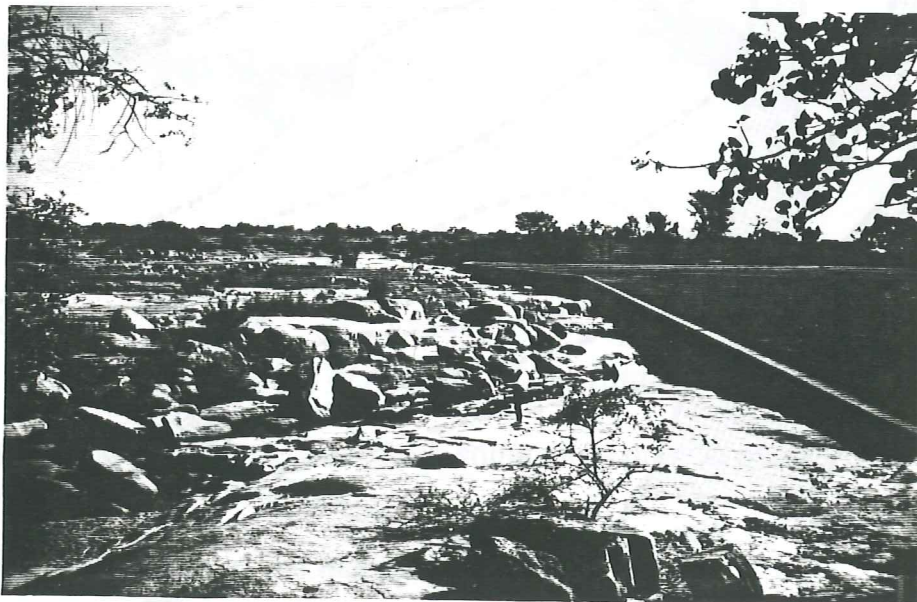
Fig 6.3.1.5 The Tuli weir and bedrock outcrops of Area 2.
