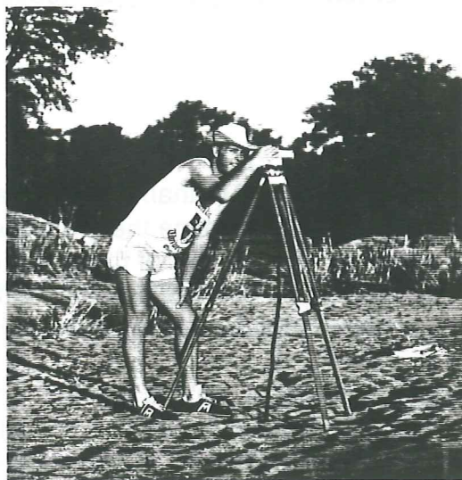
Fig 6.4.1.1 Leveling of the sand dam by Patrich.
