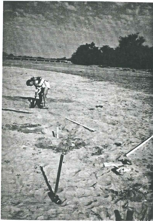
Fig 6.5.3.2 Putting groundwater pipes in position.
