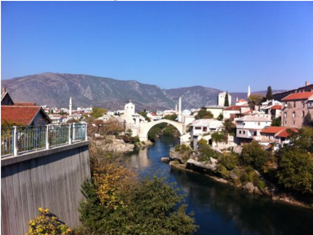
Picture 2. The rebuilt Ottoman bridge.
