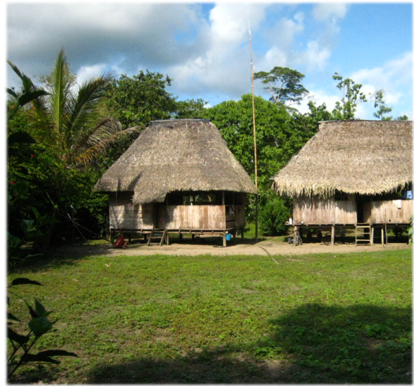
Figure 7. Traditionally built private cabins of the local inhabitants, whose design the cabins of Sani Lodge are based on.
