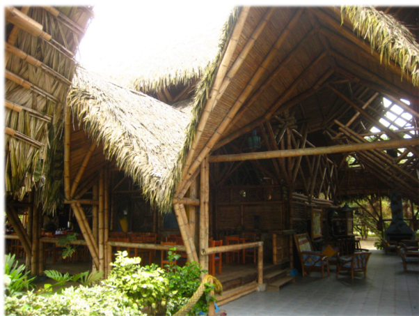
Figure 3. Some of the bamboo construction that constitutes Hostería Alándaluz and its restaurant.
