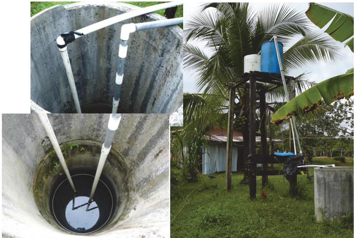
Figure 20. Private well (code A:128) used for cooking and washing.
