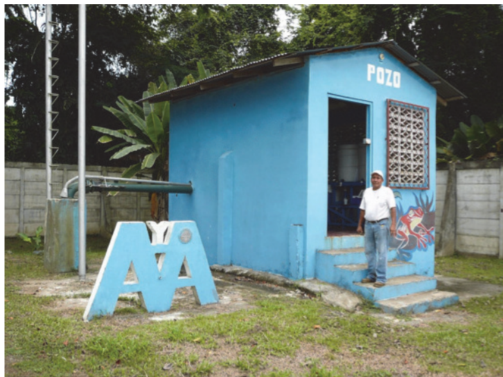
Figure 6. Well for drinking-water extraction managed by the ASADA of Venecia.
