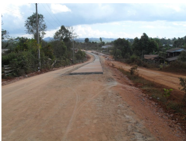
Figure 7: A new road in Galyani Vadhana District
