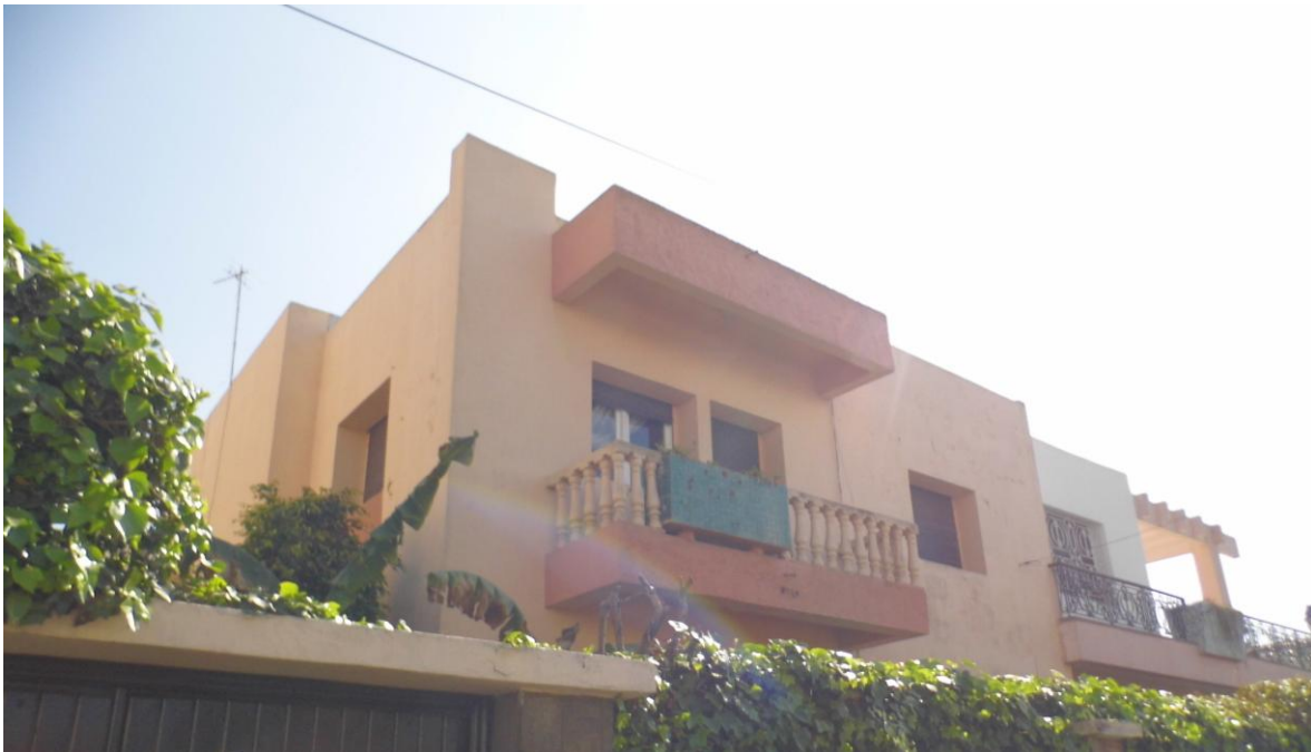
Fig 74. The house from the street, there's a wall that separates the house from the sidewalk.
