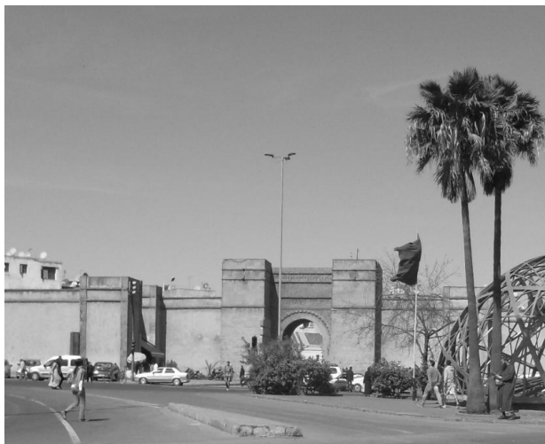
Fig 7. The main entrance in the south wall of Medina Qdima
