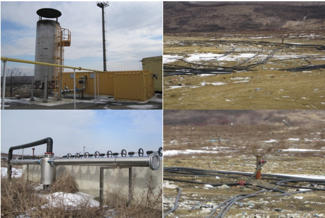
Figure 11 shows the gas collecting system at the landfill with the flare, wells and tubes (own pictures).
