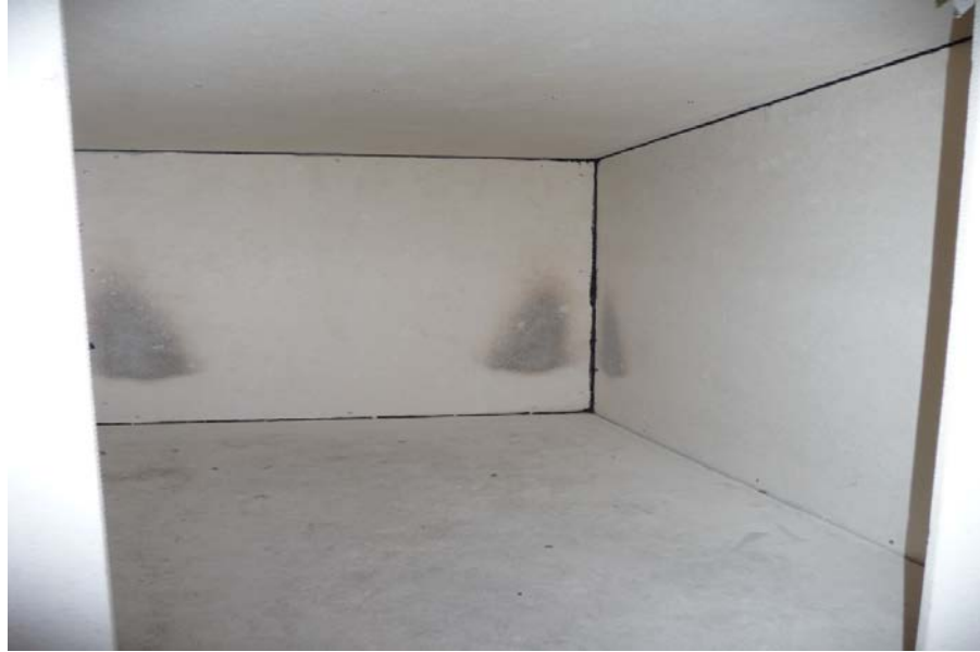
Figure 4-The room before installation and set up experimental equipment
