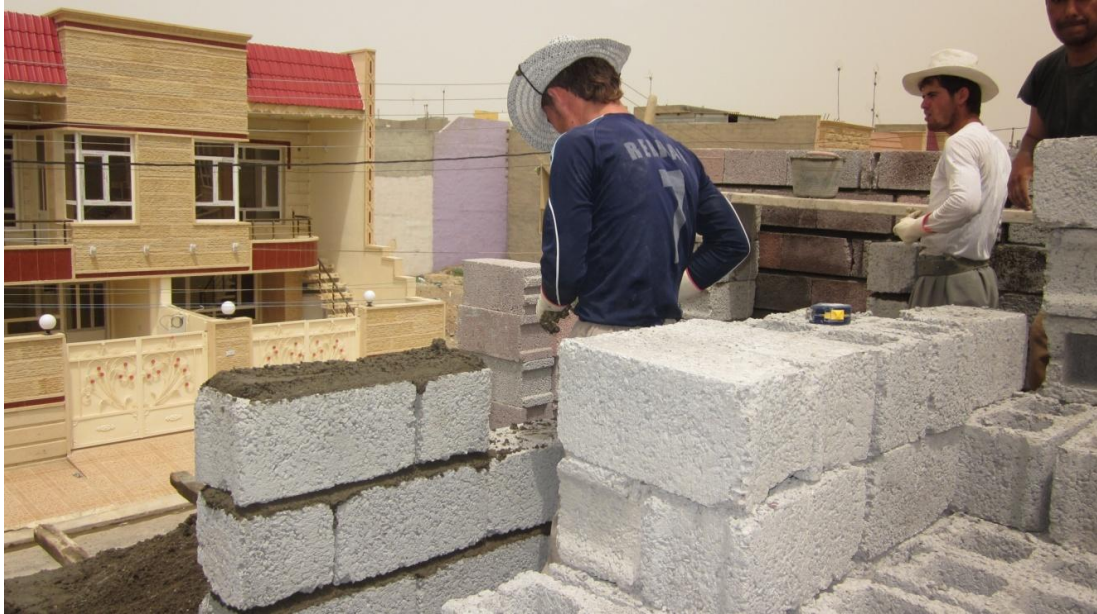
Figur 5.5 Betonghålblock
