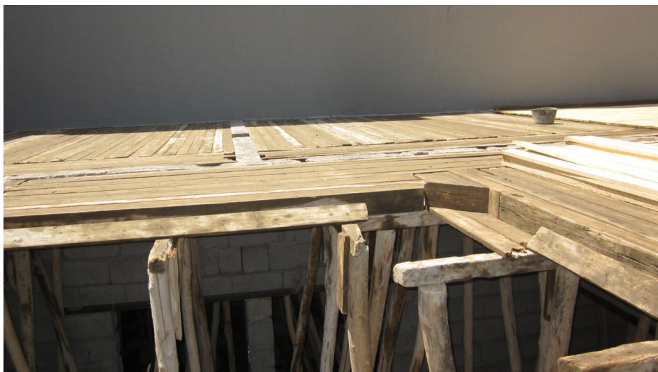
Figur 7.32 Betongbrygga (form)
