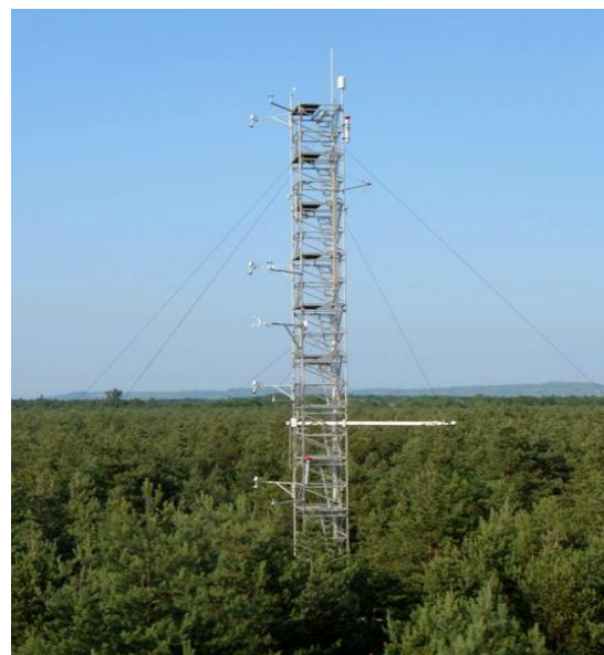
Figure 2.6: Aerial view of the experimental Hartheim forest showing the meteorological tower (Meteorological Institute, University of Freiburg)
