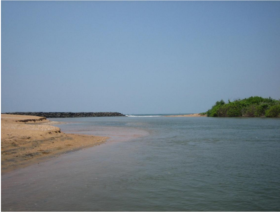
Figure 11: The Outlet at Kulamulla. In the upper part of the picture the breakwater that keeps the Outlet open can be seen.
