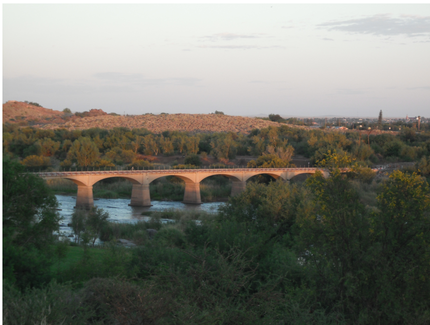
Figure 8 – Main bridge before floods (Eggers 2011)
