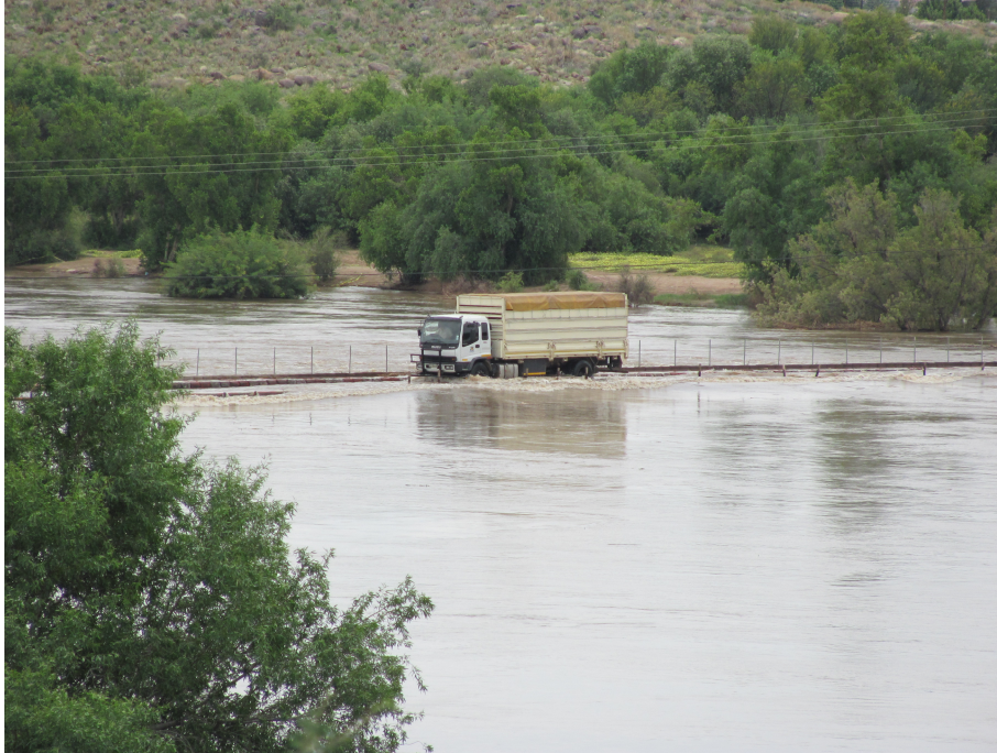
Figure 10 – Main bridge submerged, picture taken just before the bridge was shut off in January (Eggers 2011)
