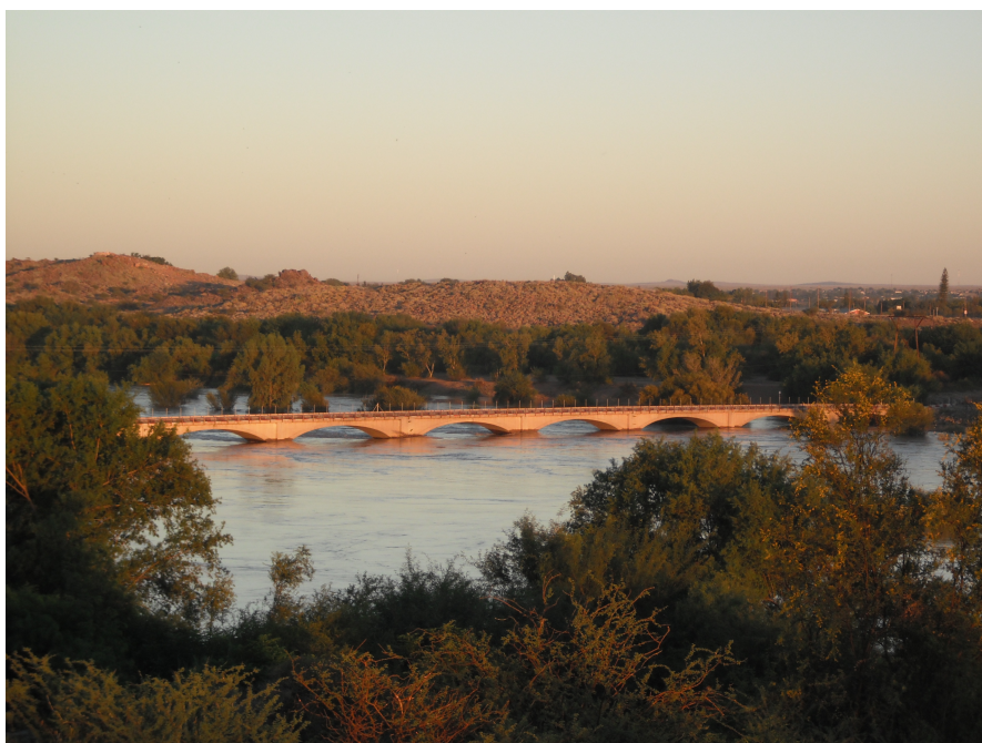
Figure 9 – Main bridge with raised water levels (Eggers 2011)
