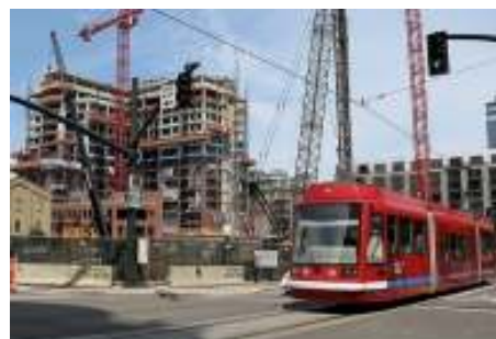
Figure 12 – Construction happening along the tramline in Portland, USA.
