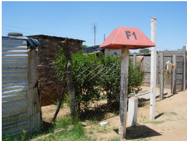
Figure 18. Sign explaining that a gas pipe was buried underneath.
