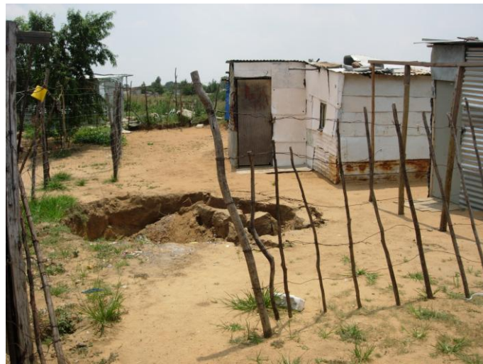
Figure 16. Sink-hole close to shacks.
