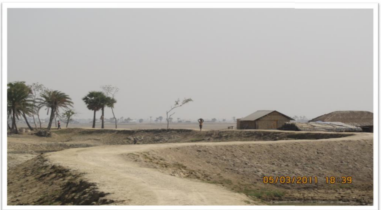
Repaied Rural Road in Dumuria
