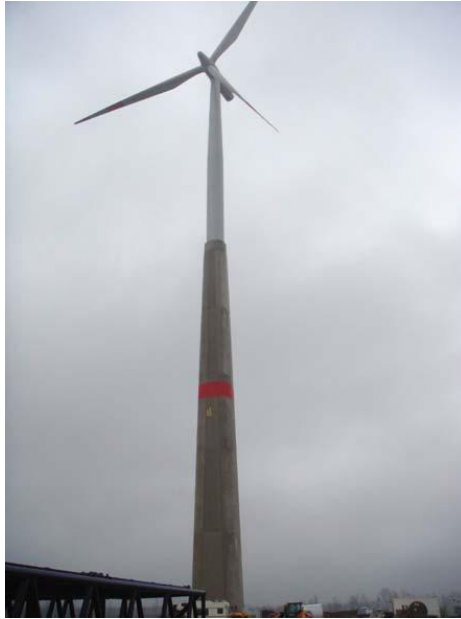
Figure 12 121 - Hybrid tower with a concrete bottom part and upper tubular steel part.
