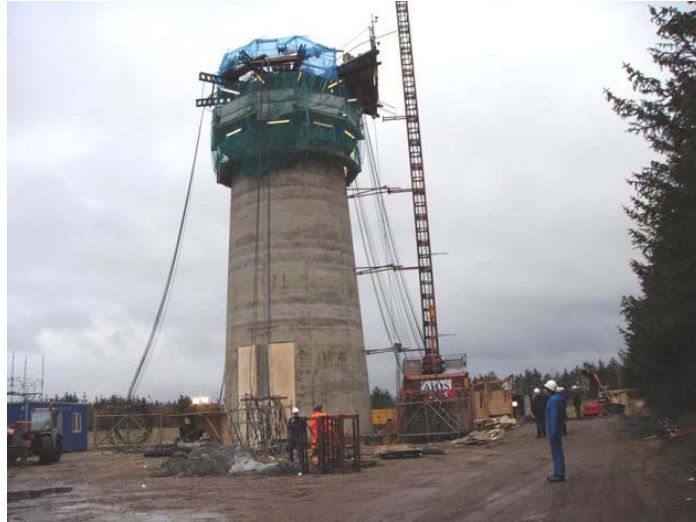
Figure 11 119 – Slip-formed cast concrete tower in production.
