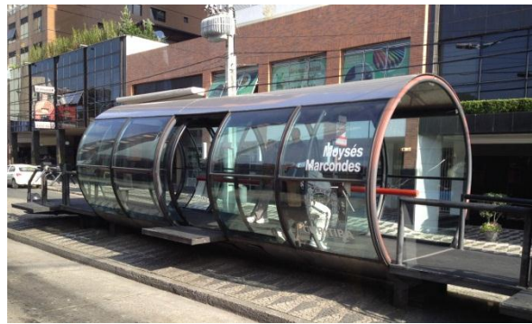
Bus station for BRT in Curitiba
