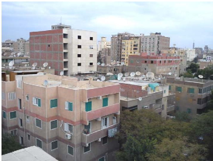
Fig. 6.5 Buildings' rooftops Dobgy Street
