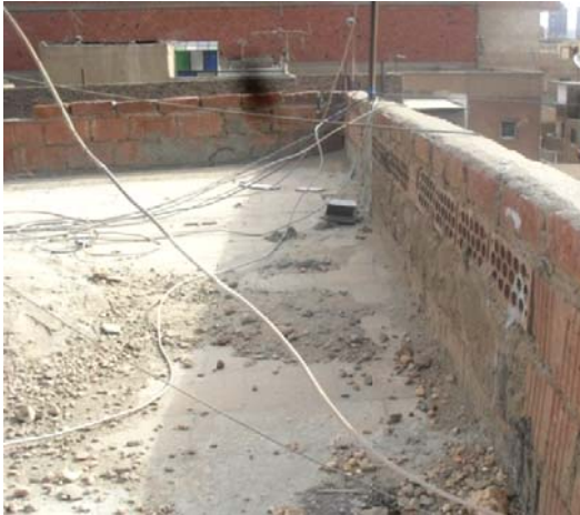
Fig. 6.4 Building #7 Dobgy Street at 10.30 am on 1 Feb 12.
