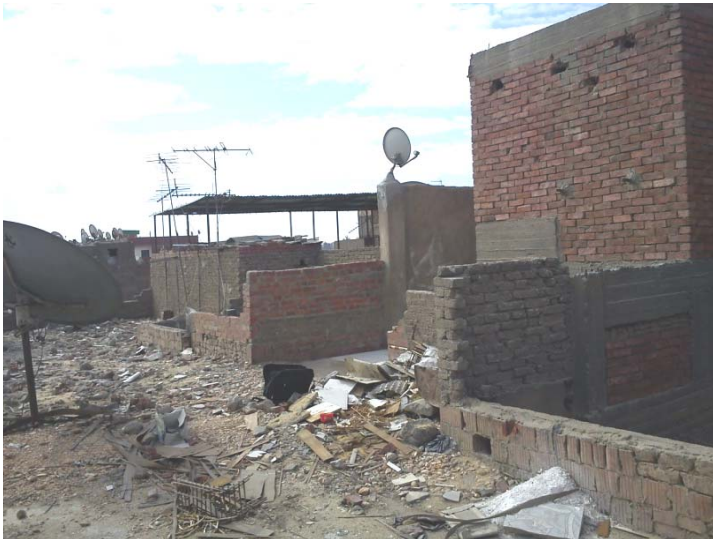
Fig. 6.7 Building # 7 Dobgy Street -Fence, dished and temp buildings
