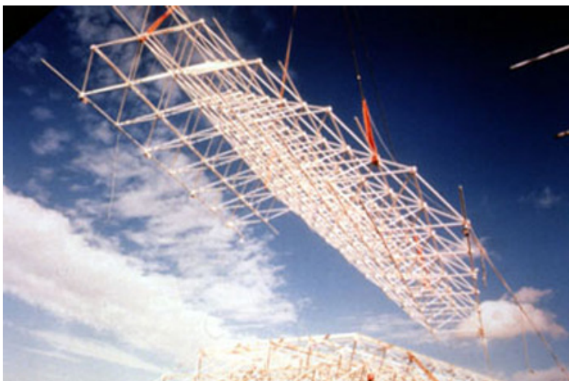
Figure 1.5.1: Erection process of the modules [3]
