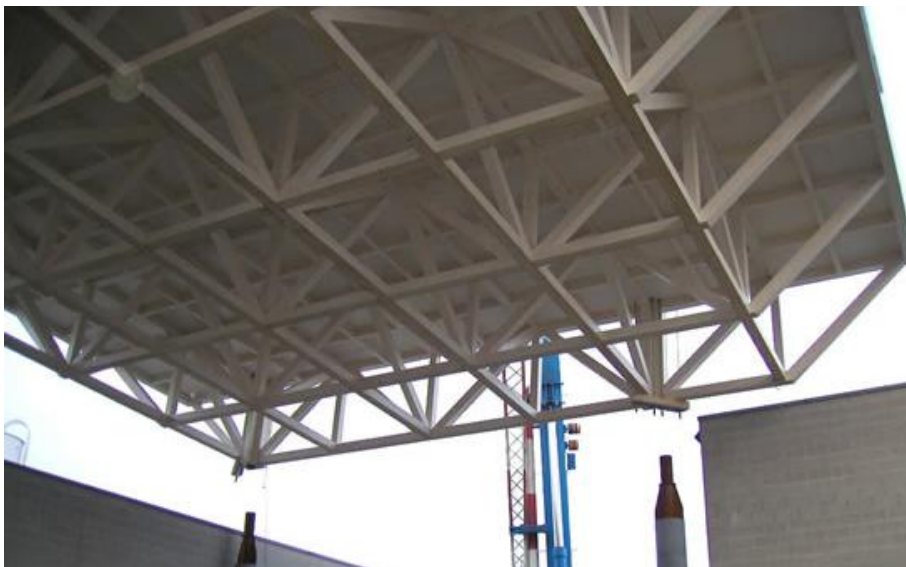
Figure 5.0.1: Glued-joint timber space structure, www.cenci.com
