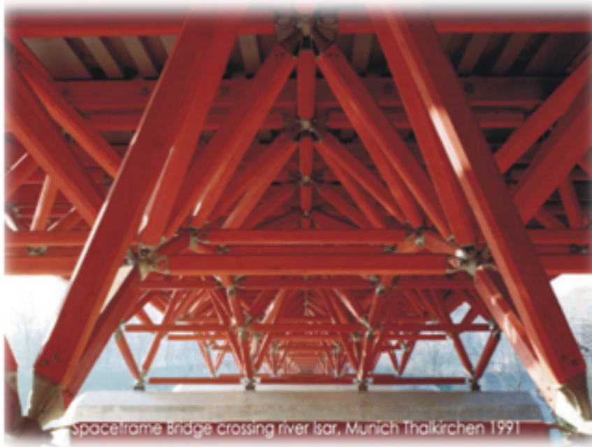
Figure 5.0.2: Dowel type joint in a space frame bridge crossing river Isar, Munich Thalrichen 1991.
