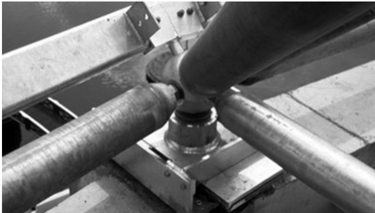
Figure 1.4.1: Lateral restraints which permits lateral deformations [3].
