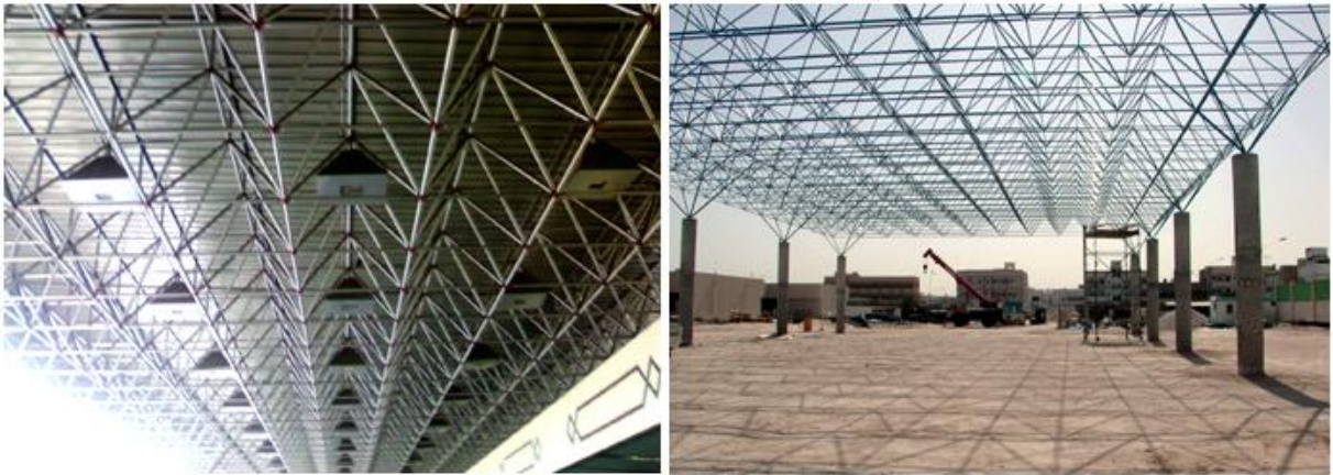
Figure 1.1.1: Flat space frame structures in India.
