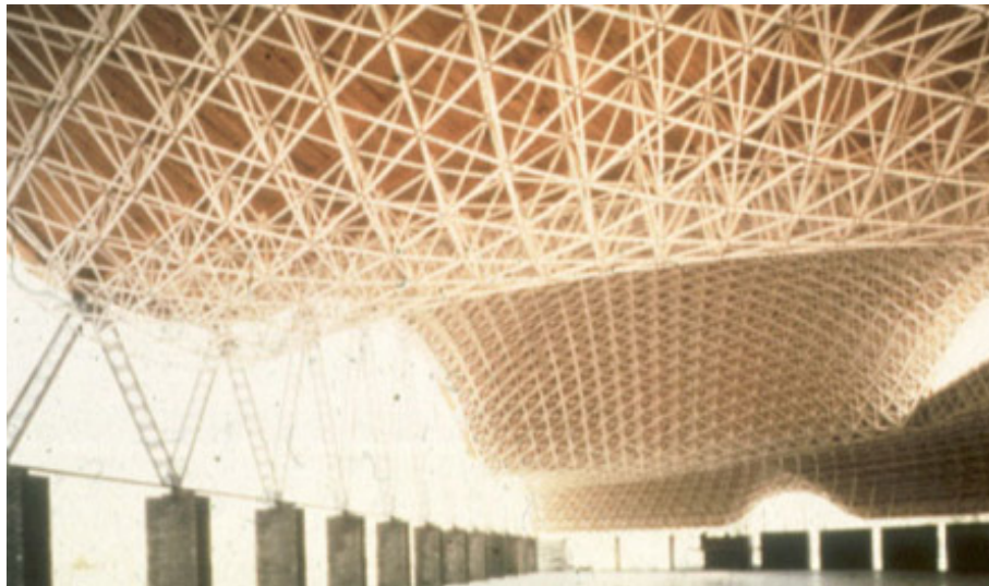
Figure 1.1.2: The roof structure of the Palafolls Sport Hall, near Barcelona, Spain demonstrates graphically that space grids do not have to be constructed as a flat plane nor to a rectangular plan [2].
