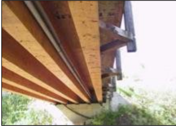
Figure 2.11 Beams protected under roadway (SETRA 2006 (2007))
