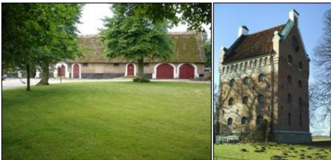
Figure 3.2 Photos of stables (left) and Börjes Tower (right)
