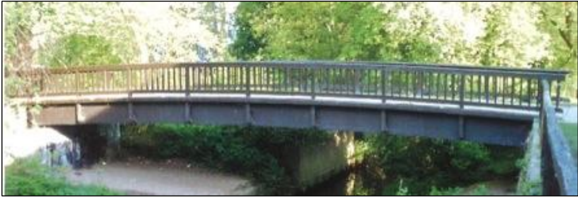
Figure 2.2 Pedestrian and cyclist bridge over the Leinbach in Heilbronn, Germany (GEROLD, M. 2007)
