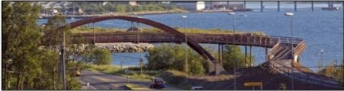
Figure 5.11 Tomasjordnes Bridge, Norway: Example of a curved bridge with a stress-laminated glulam deck (CROCETTI, R. 2012)
