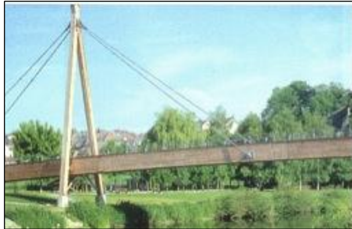
Figure 2.8 Pedestrian and cyclist cable-stayed bridge over the Lahn near Limburg, Germany (GEROLD, M. 2007)
