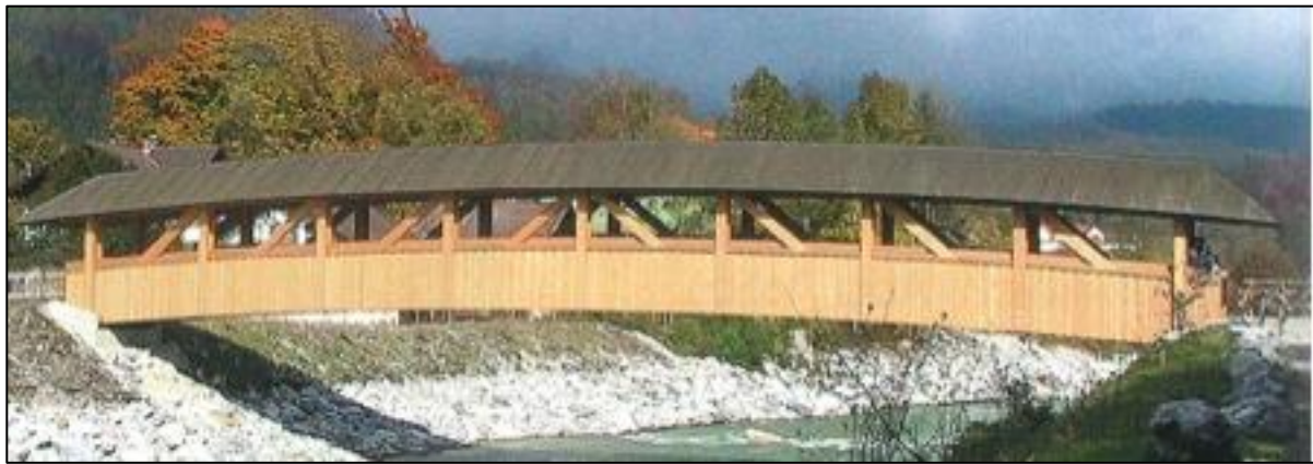
Figure 2.6 Bridge over the Loisach near Garmisch-Partenkirchen, Germany (GEROLD, M. 2007)
