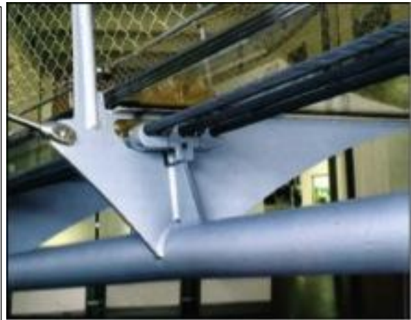
Figure 4.29 Detailed view of a diaphragm, (DEUTSCHES MUSEUM et al. 1999)
