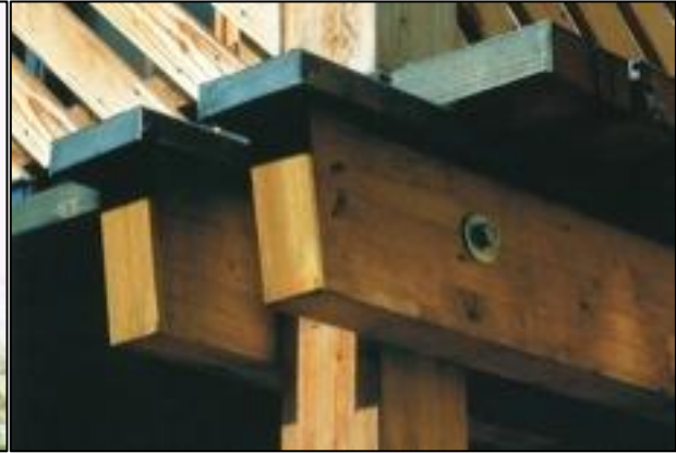
Figure 2.12 Protected horizontal beam (INFORMATIONSDIENST HOLZ 2000 (c))
