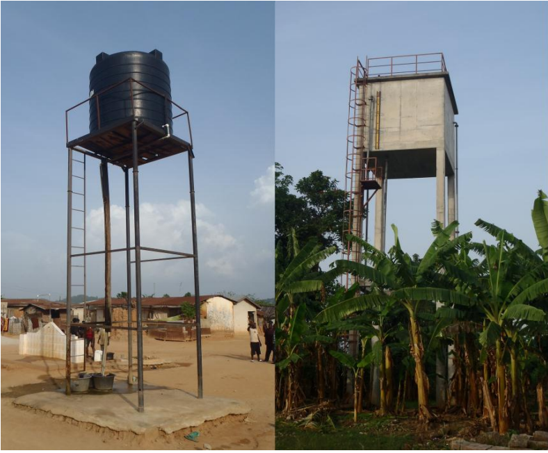
Figure 4. Plastic tank in Yaase to the left and elevated concrete reservoir in Kuntanase to the right. Photo: Kristoffer Ristinmaa
