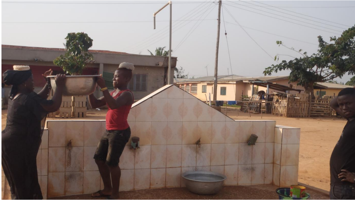
Figure 5. A stand post in Yaase with five taps including the PVC pipe that makes it possible to fetch water carrying a bowl on your head.
