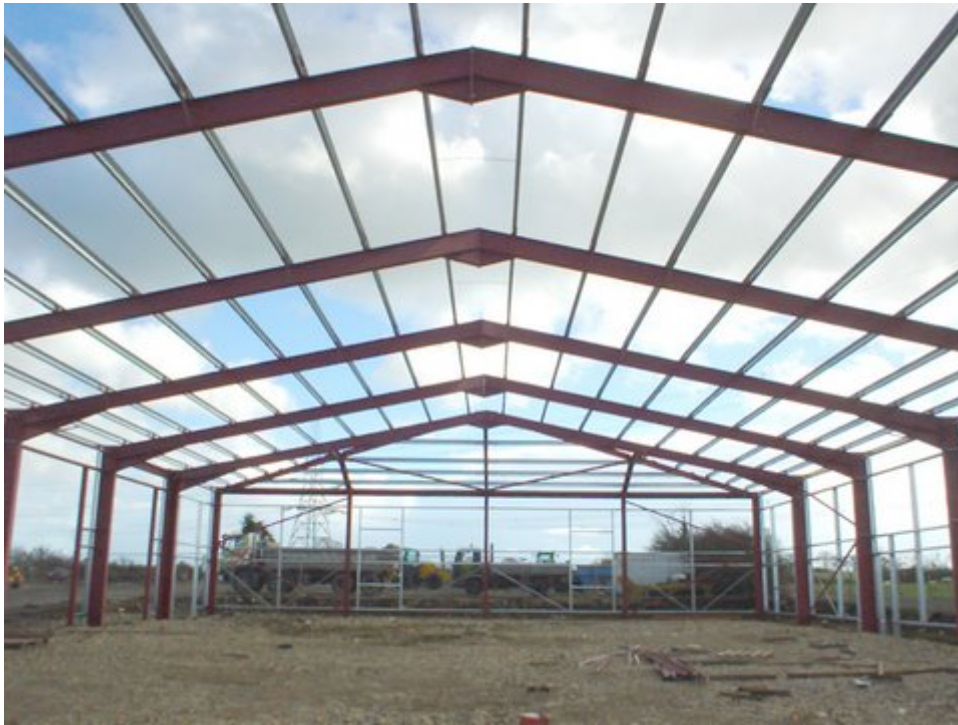
Figure 1: Steel portal frames for industrial buildings ( http://www.solid-structures.com ).
