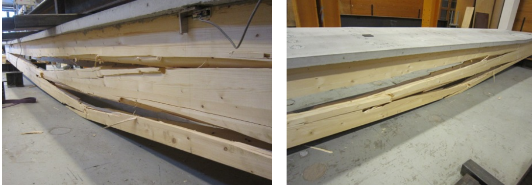
Figure 7.29: Cracks along the failed beam C2.
