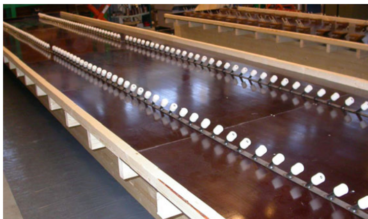
Figure 3.9: Formwork before casting of the concrete with T12 connection system.
