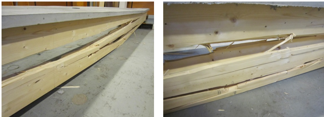
Figure 7.30: Failure of the floor system due to the sudden appearance of two cracks. It can be supposedly due to either shear or tensile stress perpendicular to the grain.
