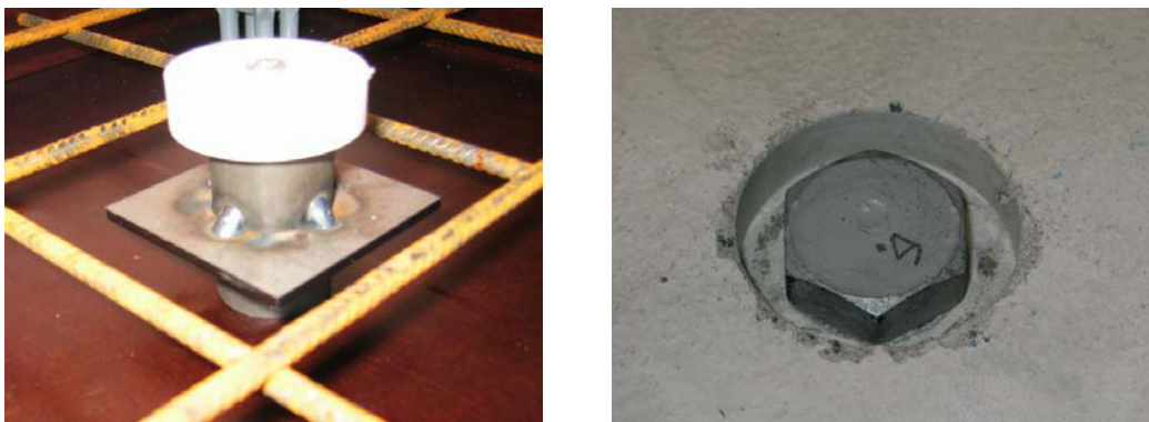
Figure 2.7: SST+S steel tube shear connectors, the moulding form with the screw's plastic cup on the left and assembled to the glulam beam on the right [1].
