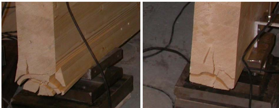
Figure 111: the timber beams start breaking for compression perpendicular to grain at the fixed support
