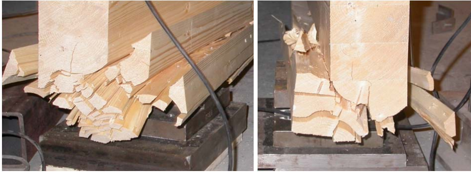
Figure 112: cross-section of the two timber beams at the fixed supports at the failure load
