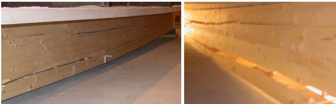
Figure 113: one of the timber beams collapsed (failure load)
