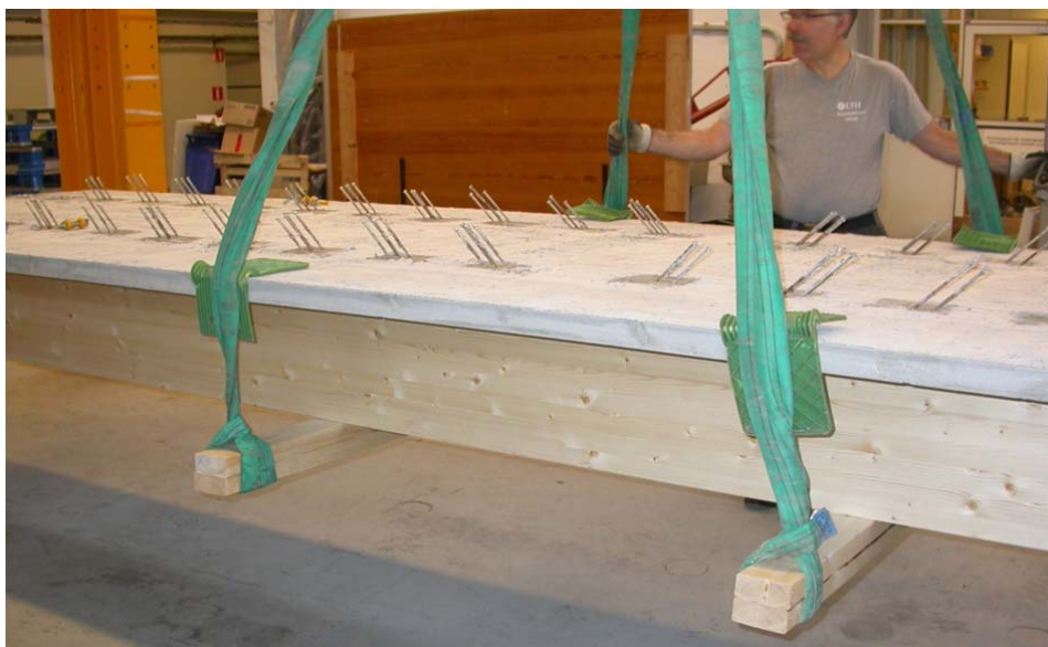
Figure 109: lifting-up of the system
