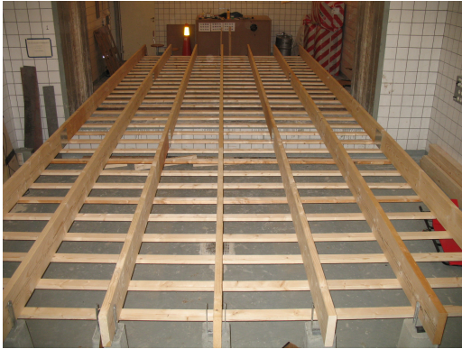
Figure 3.4: The beams with secondary spaced boarding.
