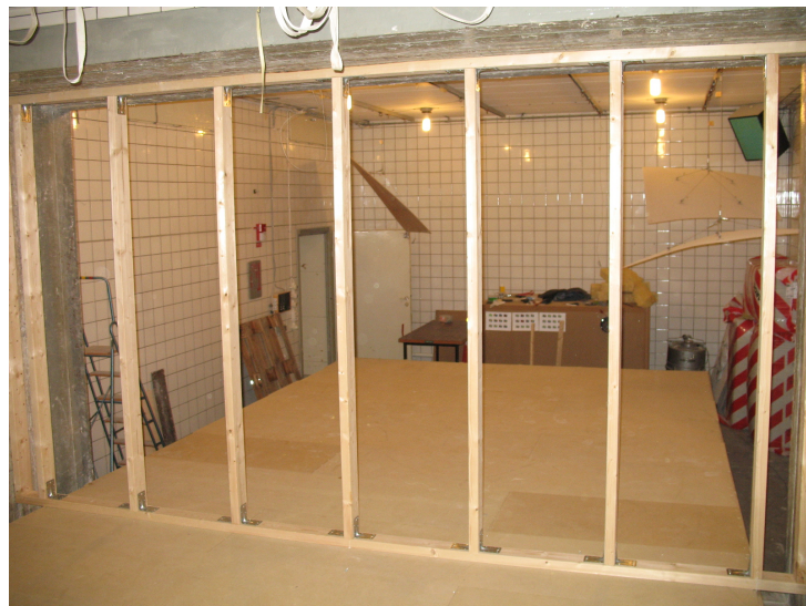
Figure 3.6: The framework of the wall.
