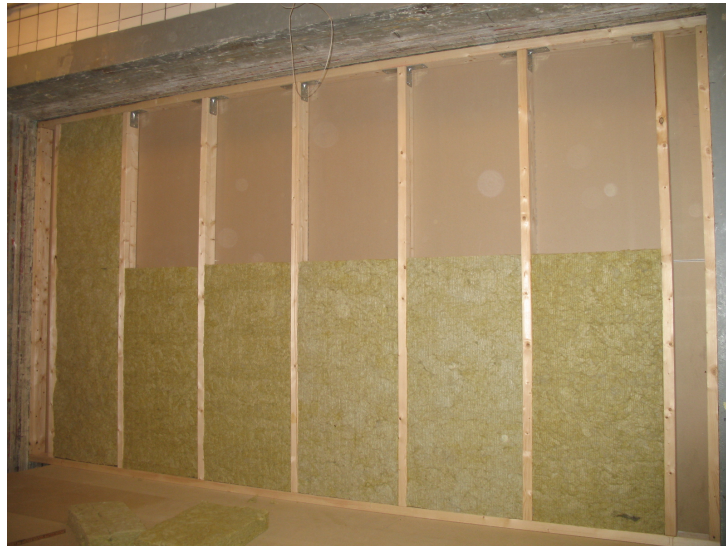
Figure 3.7: Insulation and plaster boards.
