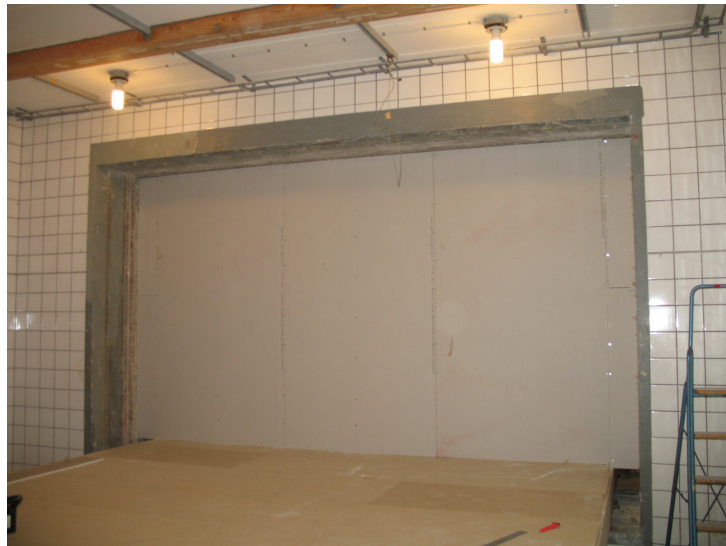
Figure 3.8: The complete structure.
