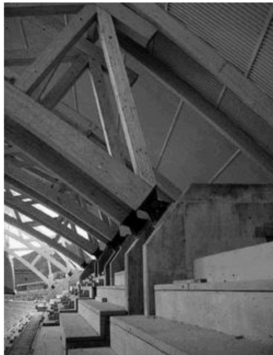
Figure 2.2. Connection joints between wooden arches and concrete foundations. (Håkons Hall, Lillehammer, Norway. Håganfang. Architect: Östgaard Arkitekter A/S. Foto: Egil Bjerke.)
