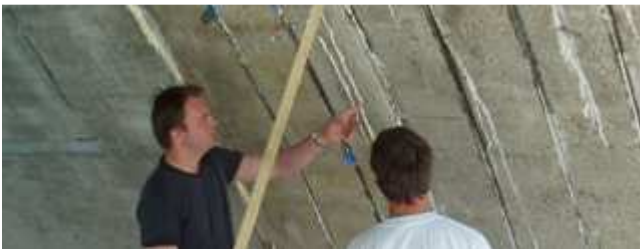
Figure 4. Application of NSMR (Sto Scandinavia AB, 2011).
