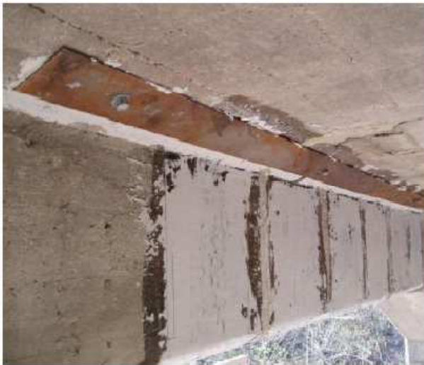
Figure 7. Mechanical anchorage with plates (Vectura, 2010).
