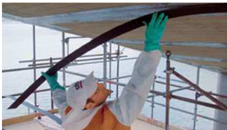
Figure 2. Application of laminate (Sto Scandinavia AB, 2011).
