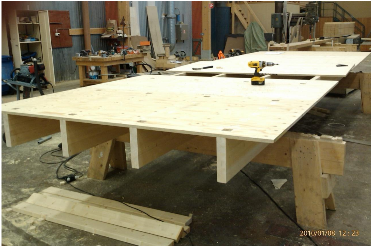
Figure D1. Manufacturing and assembling of the timber component at the Setra manufacturing Park
