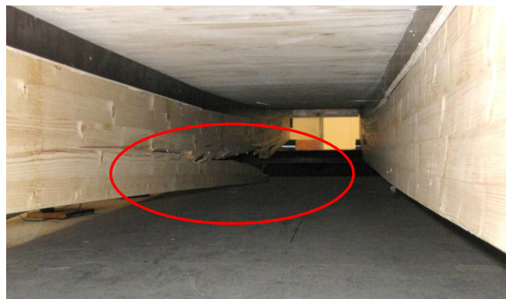
Figure 4.8 Final failure mode
