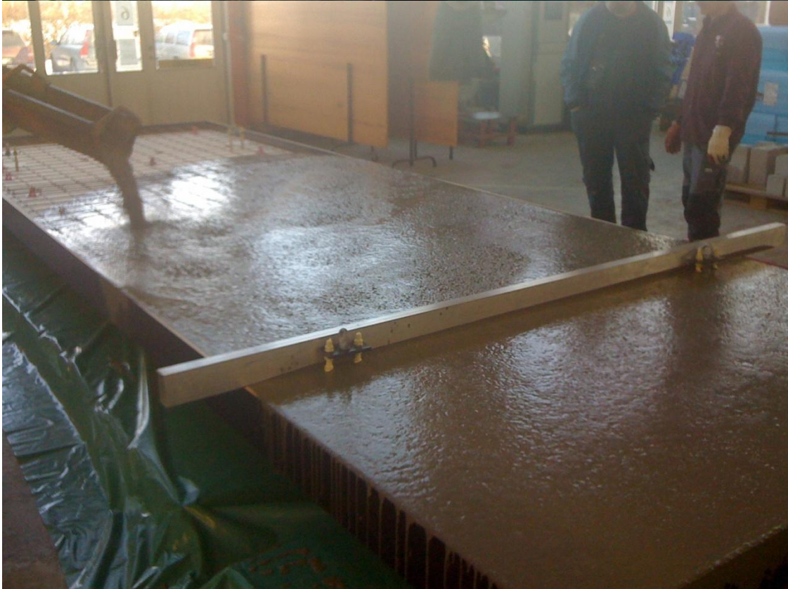
Figure D4. Casting the concrete
