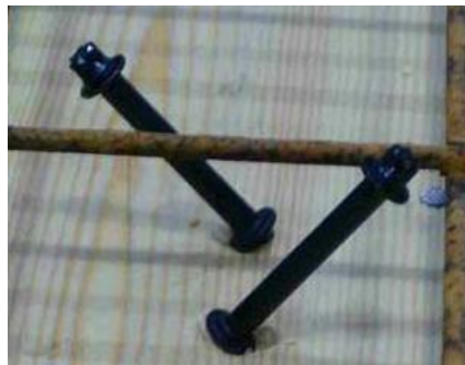
Fig 2.11 Screws installed pair-wise at angles of 45° and 135°
