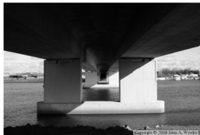
Figure 2-2: An example of a prestressed girder bridge.
