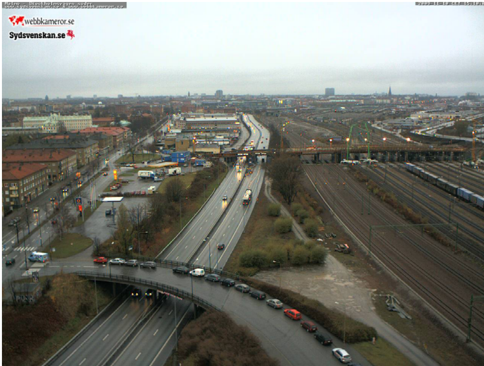
Figure 6.2 Webcam snapshot of Sjölundaviadukt during construction, seen at the top right (09-11-10 [6])
