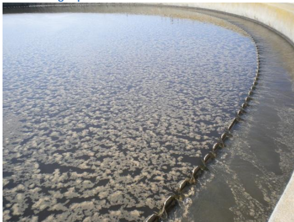
Figure 4.9. The last sedimentation and floatation is broken and the treated water contains suspended solids at SE4.
