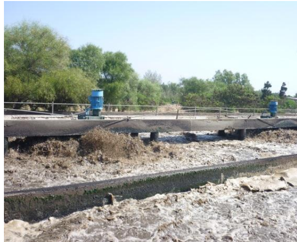
Figure 4.8. The biological treatment process at SE4.
