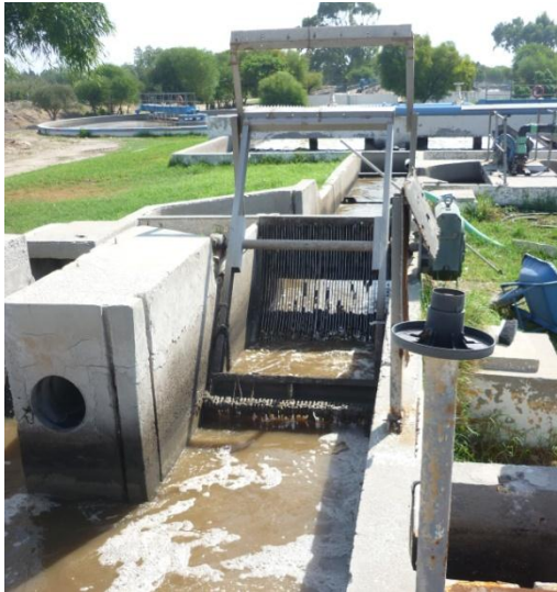
Figure 4.7. The physical treatment at SE4. This is the grid to block larger particles.
