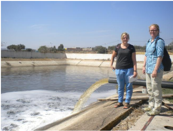
Figure 4.12. The reservoir R3 receiving water from the two wastewater plants.
