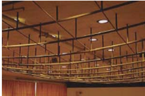
The concrete shell reinforcement hanging out in the middle
