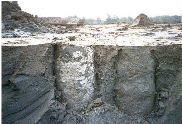
Figure 3.3: Lime/Cement columns installed in the ground [L]
