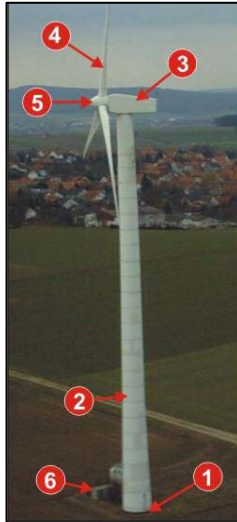
Figure 2.2: Horizontal axis wind turbine, parts numbered [D]
