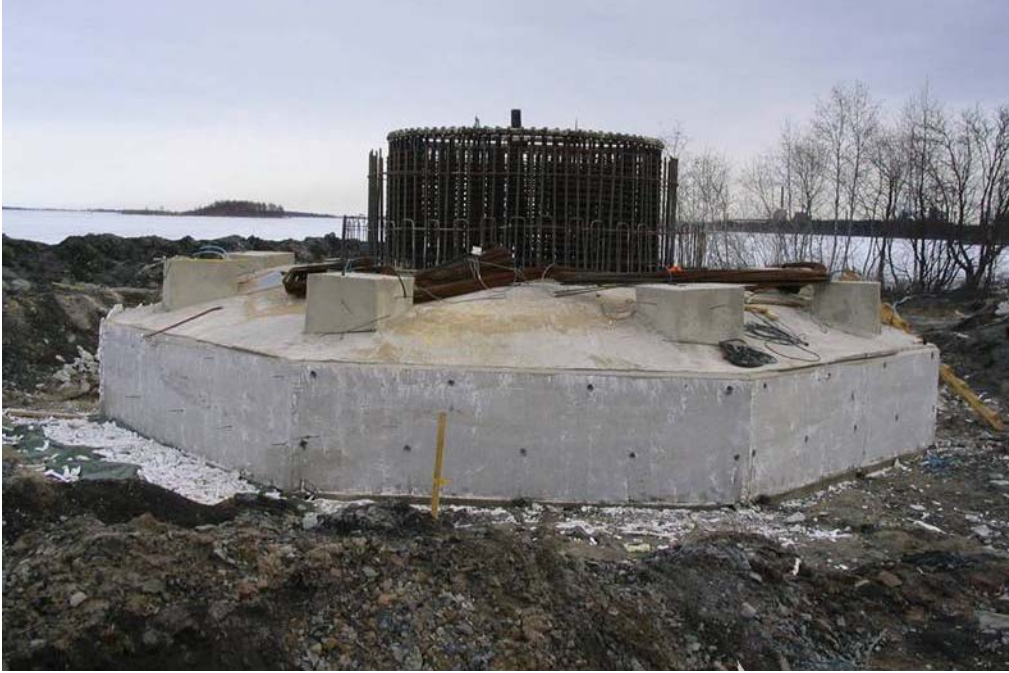
Figure 1.1: Ruukki's piled foundation [A]
