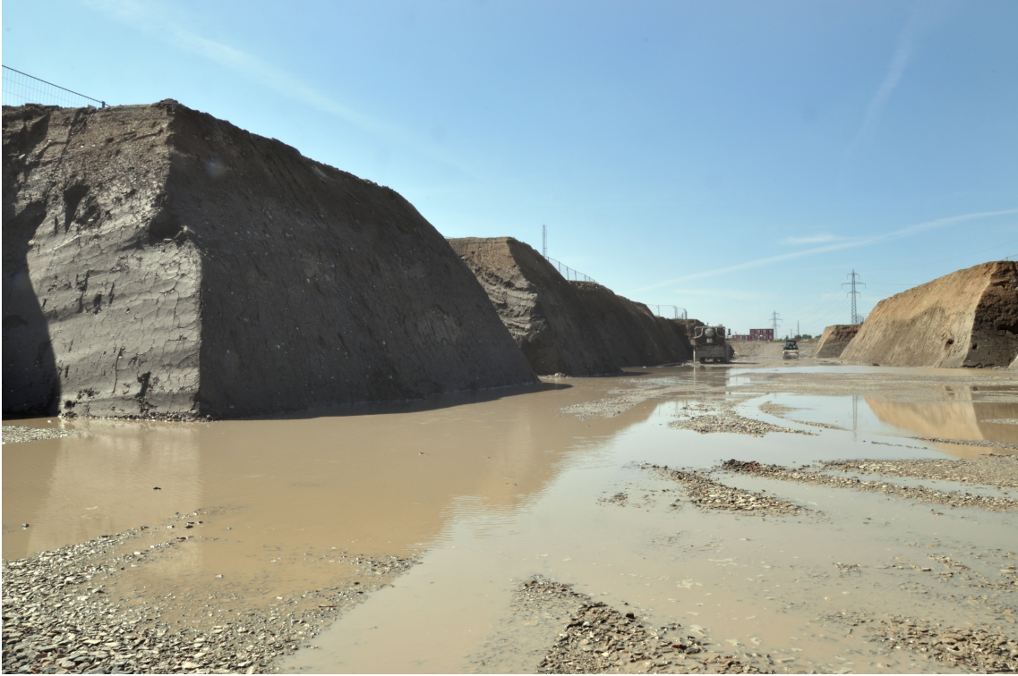
Figure 2.1: Digging of the Linac tunnel. Image courtesy of Annika Nyberg [1].
