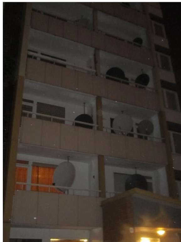
Figure 16: A building façade in Rosengård. Every apartment has its own satellite dish; may imply they watch program in their own language and culture that can impede increasing their knowledge about their host society.
