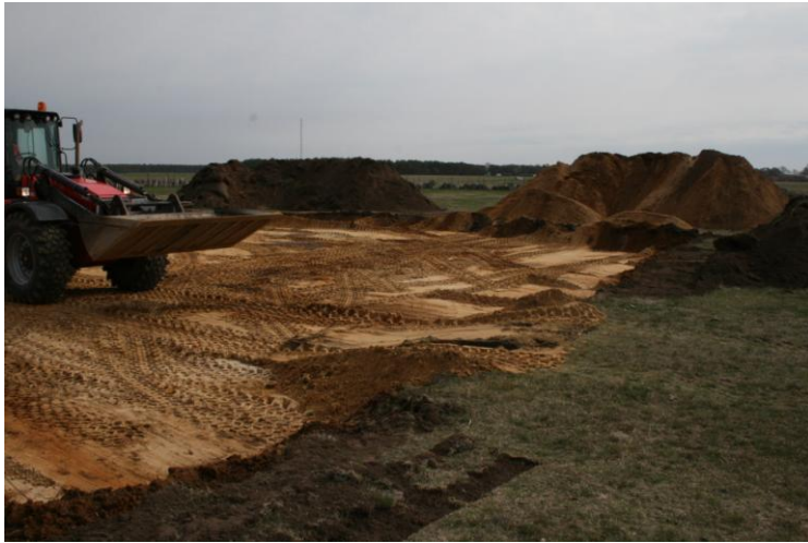
Fig. 6 Backhoe loader doing soil perturbation at Ripa 1-3.
