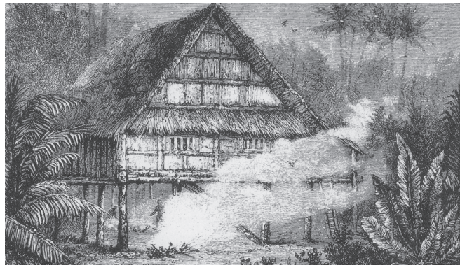
Pile- built house with slatter floor, burying trash and smoking the mosquitoes away (Waterson, 1997, p. 89).
