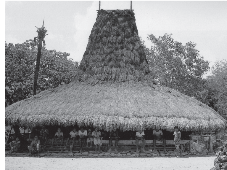
Traditional house, West Sumatra. The roof is built on a truss and crossbeam structure, and traditionally thatched with ijuk, palm fibre, lasts up to 100 years. PHOTO: Roxana Waterson (Waterson, 1997, p. 77)
