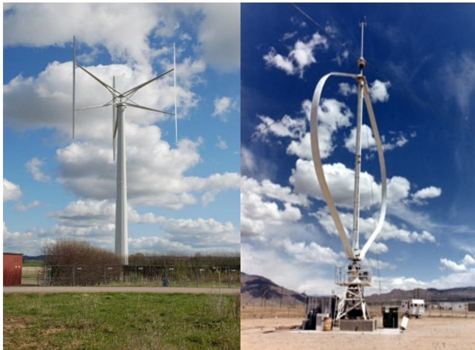
(a) Giromill design of a VAWT placed in Falkenberg, Sweden [5] (b) Darrieus design of a VAWT [6]
