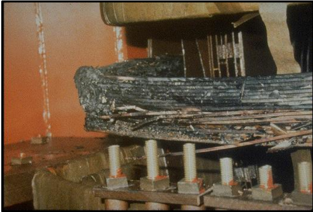
Figure 5: Close-up view of a part of the transformer that was damaged at the Salem Nuclear Power Plant (courtesy of Peter Balma).
