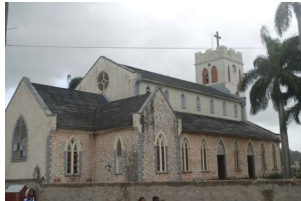
Figure 6: The parish church - still used today for services
