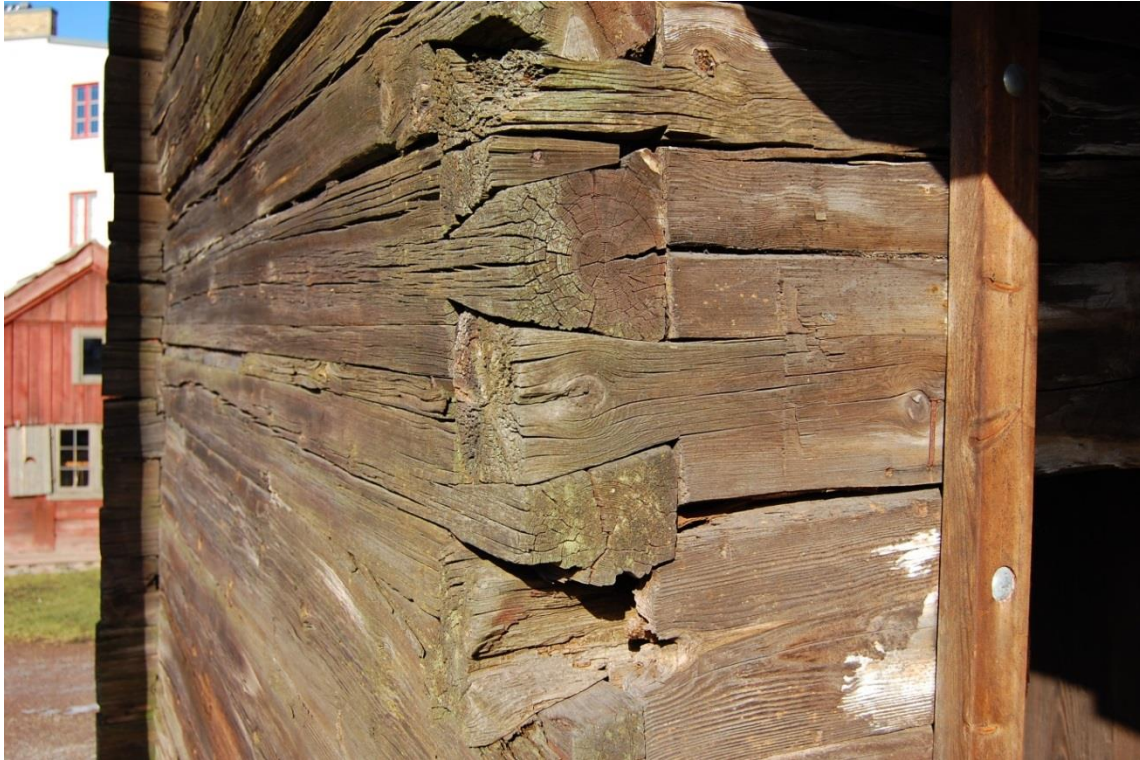
Figure 6. The “hen house” corner on the front of the house. The technique used is the corner timber . The picture shows the cut in the logs used to connect the end of the trunks. To the left of the picture it is possible to see the far end of the logs extruding from the wall. (Picture: Linda Nesi, 2013).
