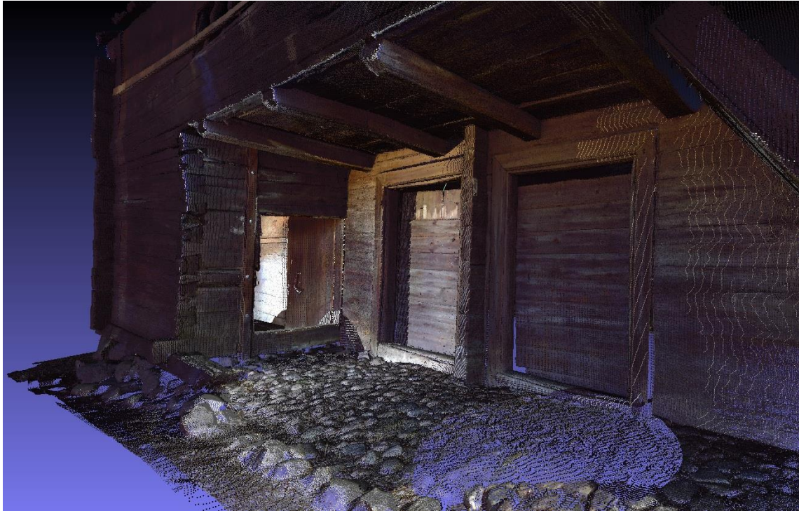
Figure 8. Screenshot of the point cloud showing the area scanned under the gallery and the “hen house”. Three scans (12, 13 and 14) have been performed to cover this part, as showed in figure 11.
