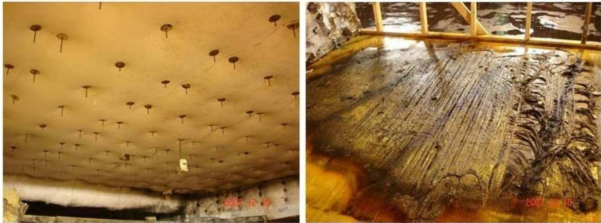
Figure 15. Overhead deck's bottom side and cabin floor, after completed test (Hertzberg, Axelsson, & Arvidson, 2008).
