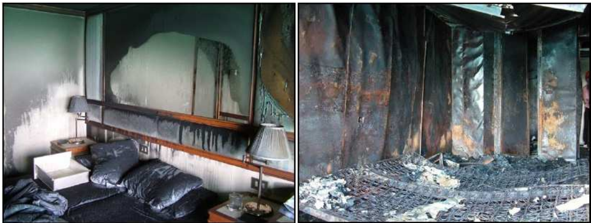
Figure 22. Damage done to a cabin with a functioning hi-fog system (left), and damage to the cabin with a malfunctioning hi-fog system (right) (MAIB, 2006).
