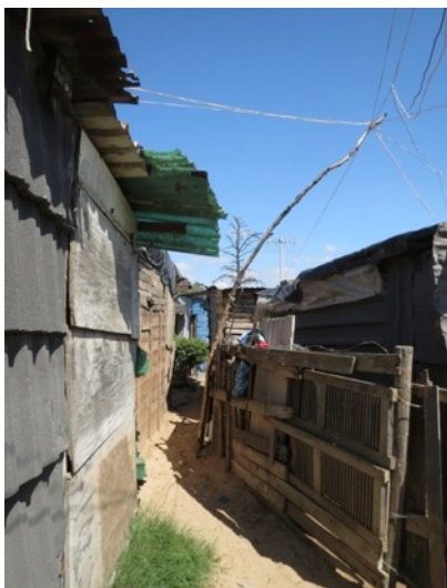
Figure B5. Narrow walking paths and inappropriate usage of electricity cables.
