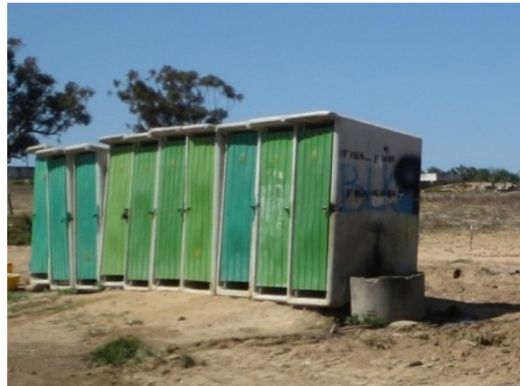
Figure B4. Toilets.
