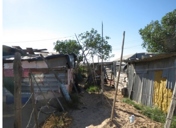
Figure B2. Poorly constructed dwellings.
