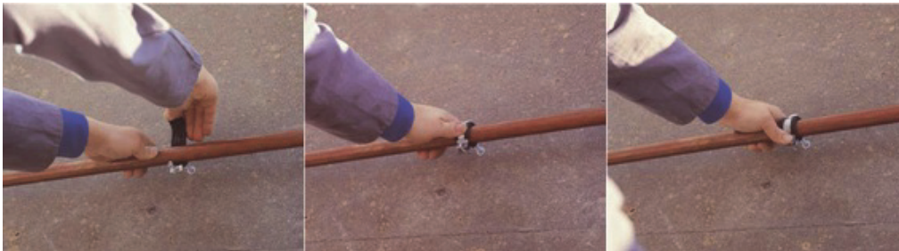
Figure 11: Using tube clamps.
